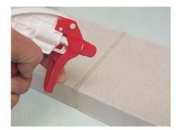
Step 8. Spray the joint with a fine mist of water to prevent the mix drying too quickly. Protect the areas in adverse conditions by covering with plastic sheet.
