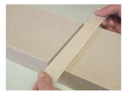
Step 4. Prepare the joint to be pointed by masking around the joint. This will prevent any excess pointing mix from staining the surrounding stone.
