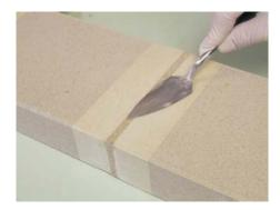
Step 6. Once the joint is full, smooth the surface of the pointing mix flush with the surrounding stonework.
