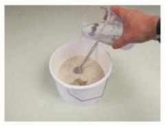
Step 2. Once the dry ingredients are thoroughly mixed, add the water in small quantities and mix well. Only mix the required amount that can be used within one hour.
