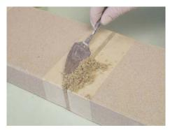
Step 5. Using the small pointing trowel, fill the area required compressing the mix well into the joint
